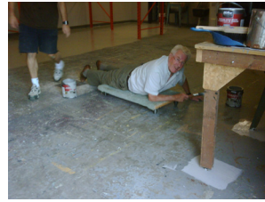
(A) Tony Francis, hard at work painting the workshop floor. Photo: Jim Clarke.
