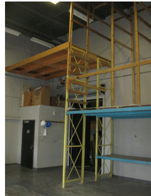
(A) The workshop, before and after the "extreme makeover". Photos: Jim Holmes.
